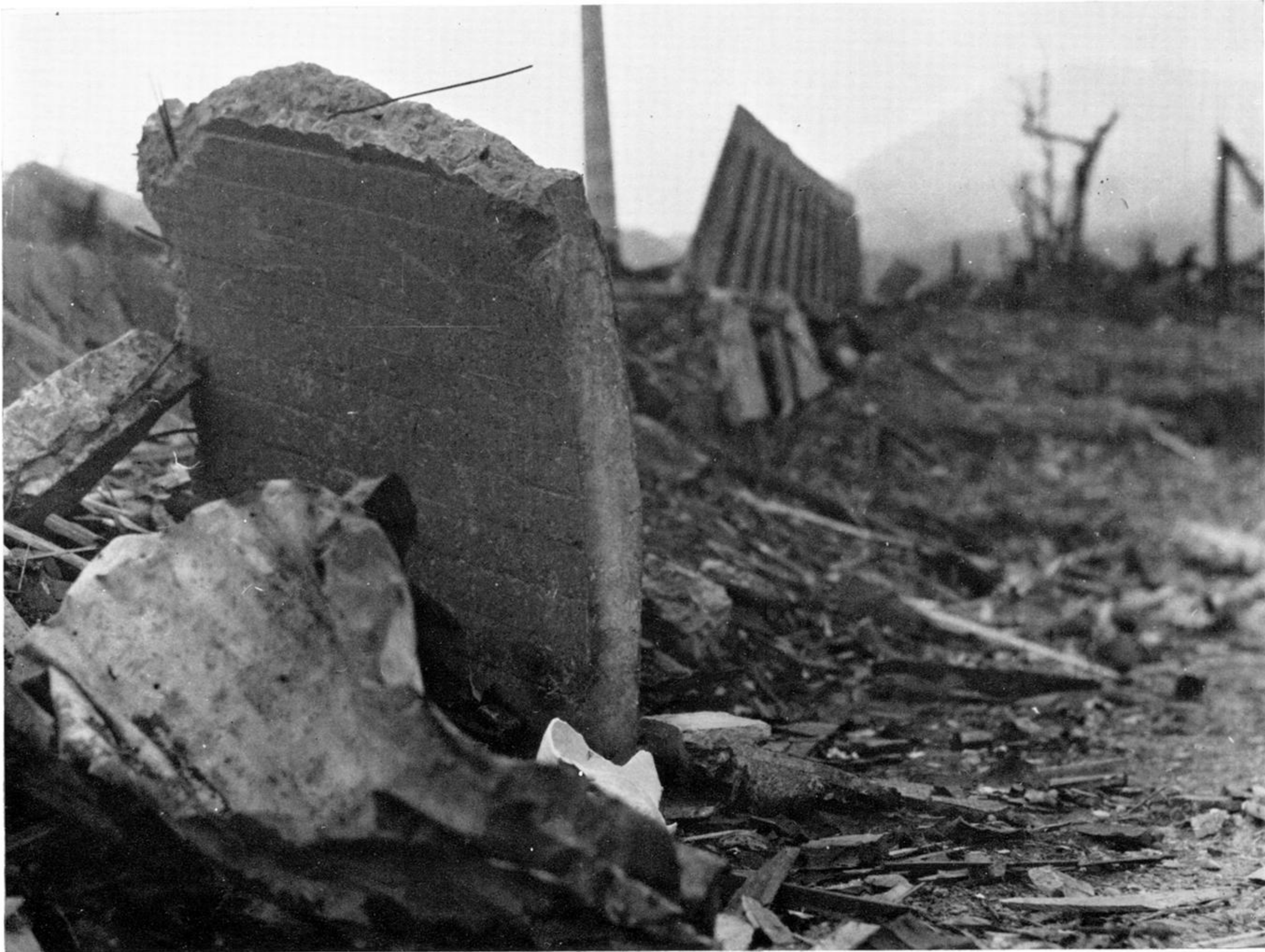
FIGURE 20. A piece from the top of the wall around the prisoners of war camp in Nagasaki thrown by the blast.
