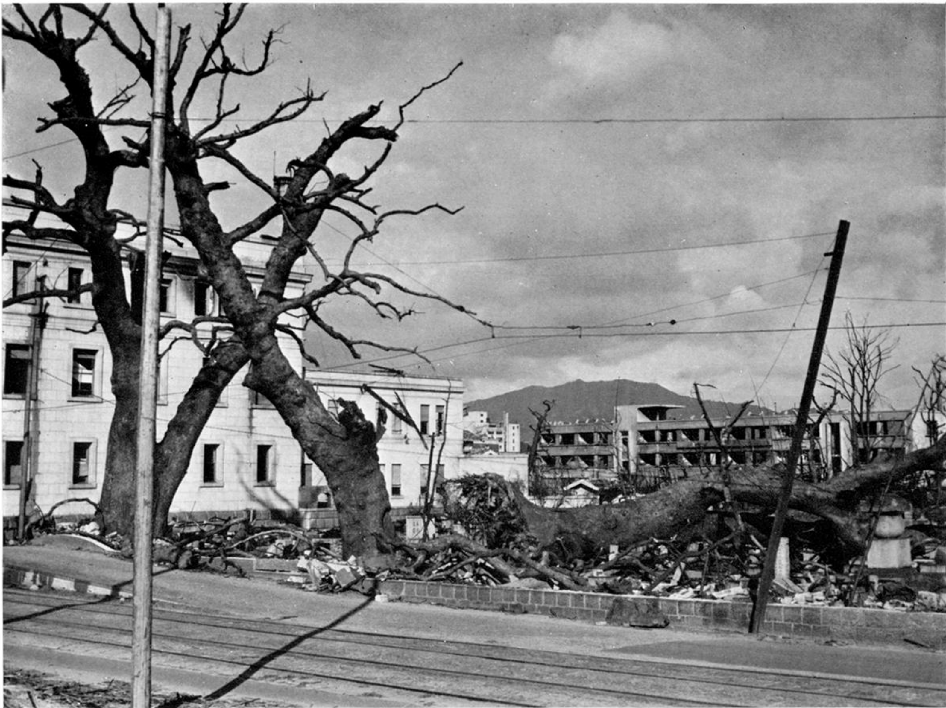
FIGURE 14. A power line pole which did not break, an I beam power line support pole which bent and an uprooted tree near the Appeal Courts in Hiroshima.
