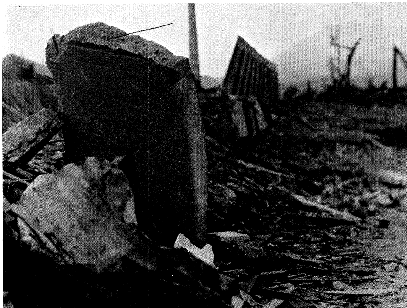
FIGURE 20. A piece from the top of the wall around the prisoners of war camp in Nagasaki thrown by the blast.
