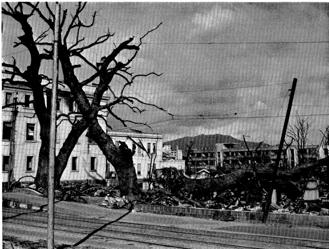
FIGURE 14. A power line pole which did not break, an I beam power line support pole which bent and an uprooted tree near the Appeal Courts in Hiroshima.
