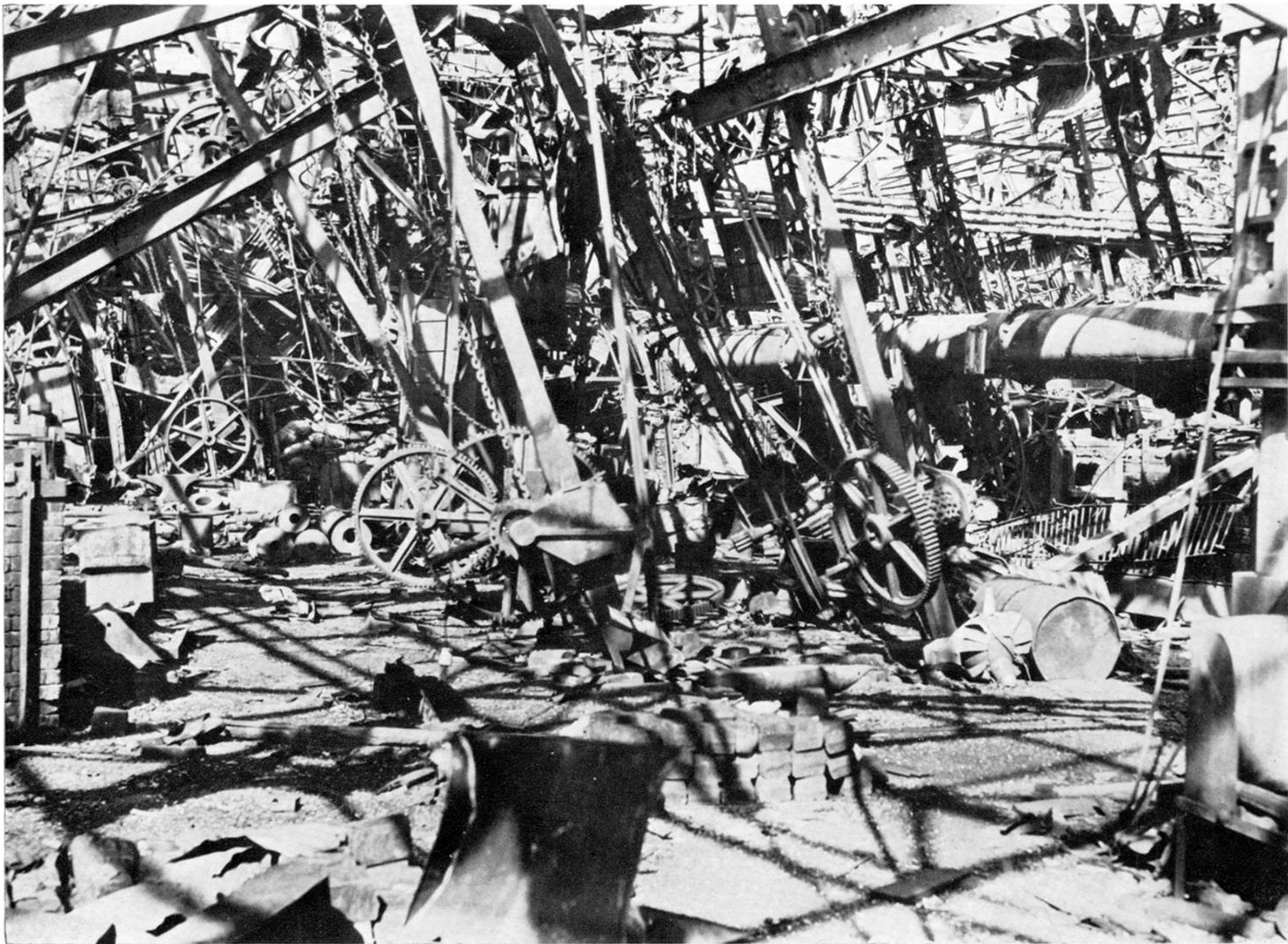
FIGURE 32. A thin wall empty can with filler cap missing, collapsed by the blast at Nagasaki. The 46-gal drum was full of water.
